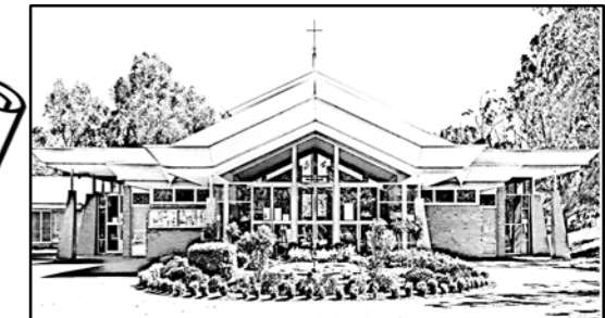
St Michael's Church Tyrrell Cct Kaleen
